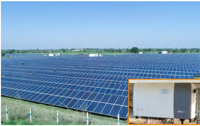
Soleos Energy Project, India 2MW
