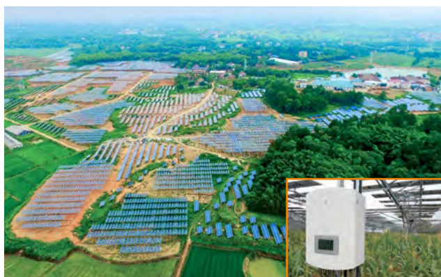
Zhejiang Quzhou Agricultural-photovoltaic hybrid PV plant 20MW
