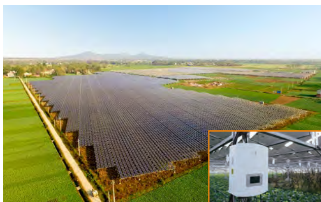
Hubei Guanyin Agricultural-photovoltaic hybrid PV plant 20MW
